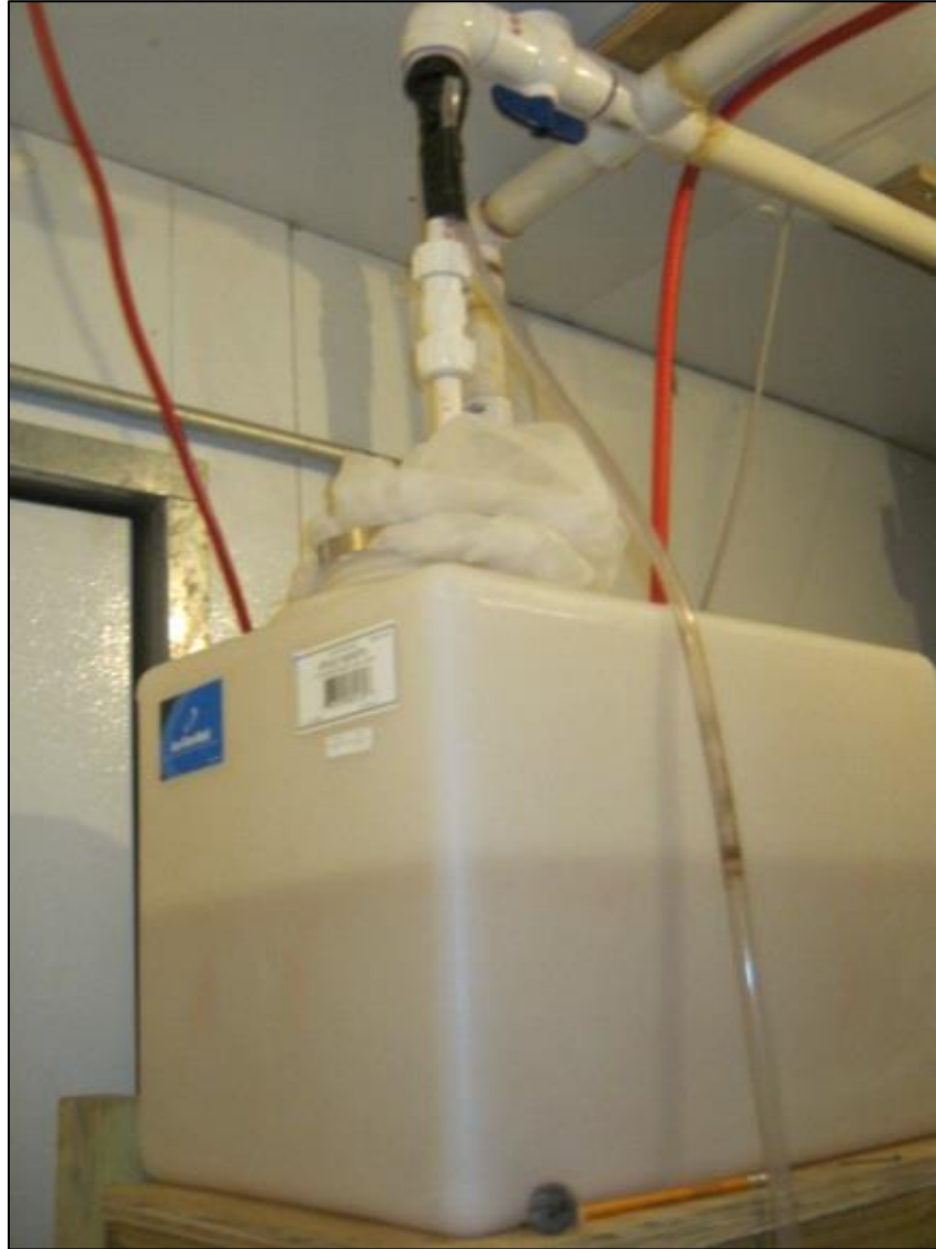
Figure A3. An image of the influent piping system and dose tank.
