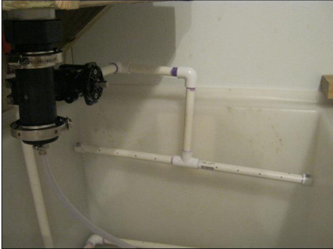
Figure A5. An image of the influent manifold (PVC pipe) before the addition of pea gravel.
